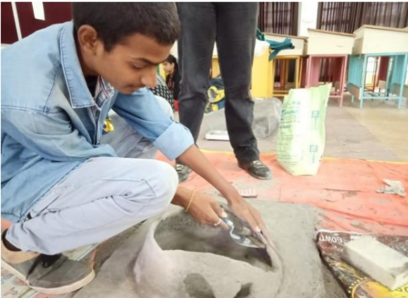
3rd year students working on the plastering of the ferro cement model on 15-09-2019 @E210 - School of Architecture
