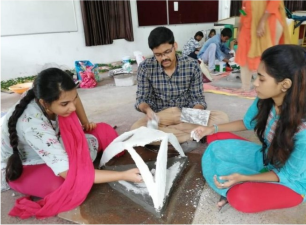
3rd year students working on the plastering of the ferrocement model on 15-09-2019 @E210 - School of Architecture
